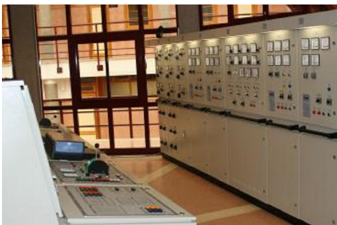
Fig. 2 MED3DH– Switchboard panels
