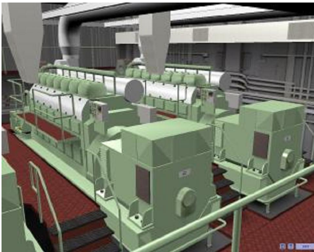
Fig. 7 MED3DH - Auxiliary Diesel Generators - 3D view
