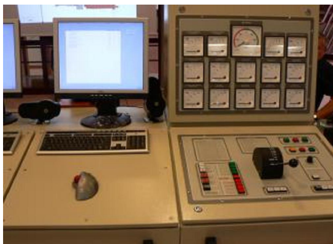
Fig. 20 ERC 4.5 XL Main Engine Control Panel.
