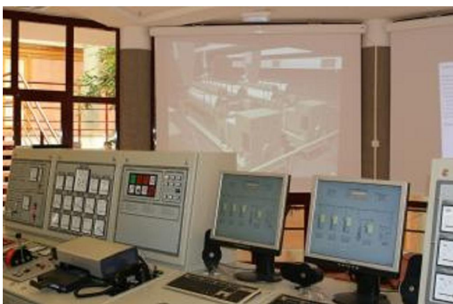
Fig. 3 MED3DH - Engine control room consoles
