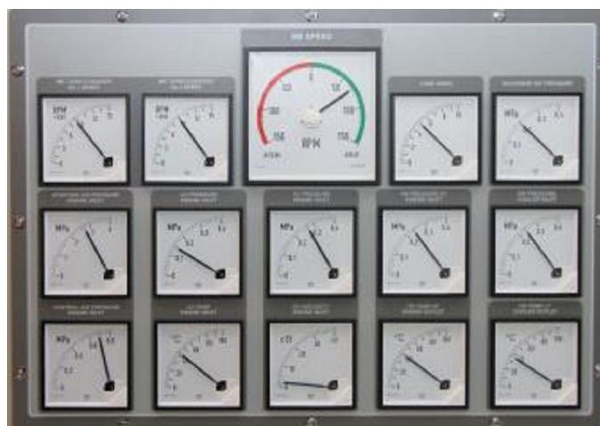
Fig. 22 ERC 4.5 XL Main Engine Control Console upper part.
